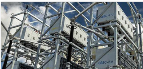
N. GRID SUBSTATION UPGRADE, HARKER £250m
